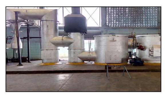
The effluent generated from scrubbing mechanism shall be properly treated in Effluent Treatment Plant and can be used in the alkaline scrubbing mechanism.
